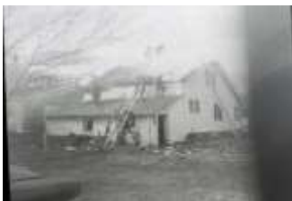
Center Line House Fire
