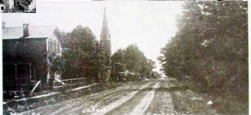
Main Street. (Van Dyke) Center Line. Steeple of the new church built in 1880 can be seen.
