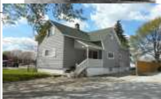
J Kaltz House
